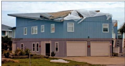
success can be overshadowed by poor design, construction, or maintenance. The North Carolina house shown in Figure 4-4 was set back from the shoreline and safe from long-term erosion, but, it could not resist winds from Hurricane Floyd in 1999.
