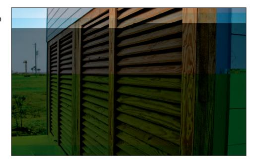
Figure 2-22. An enclosure formed by open lattice (Isle of Palms, SC)
